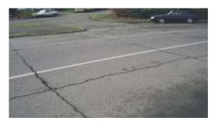
The most common *causative* agents of this type of cracking are due to joints and cracks in the pavement layer underneath.
