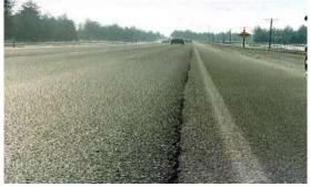
The possible <u>causes</u> include poor drainage, shoulder settlement, weak joints between adjoining spread of pavement layers or differential frost heave.
