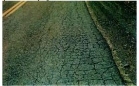
The possible <u>causes</u> include inadequate structural support which can be caused by a number of things. A few of the more common ones are listed here;
